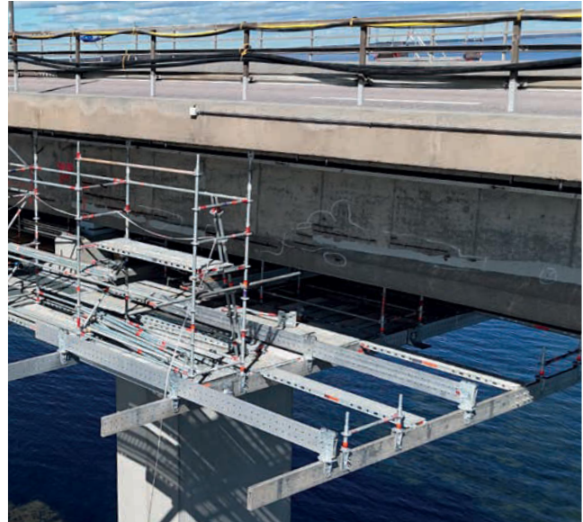
FlexDeck work platform assembled using a cantilevered construction method underneath a bridge (assembled condition shown)
